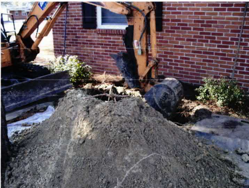
Picture 2: UST 804Azalea excavation in progress.
